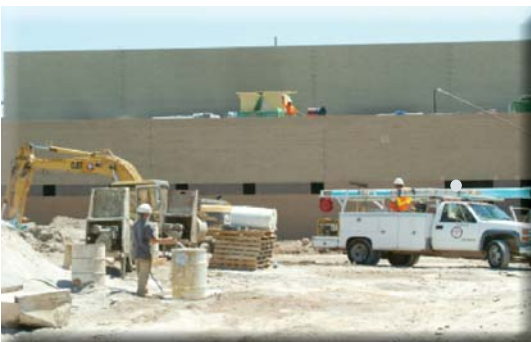
New school being built under the watchful eye of a CCSD building inspector.
