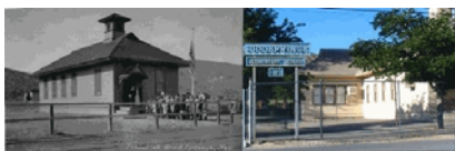
L-R: Goodsprings Elementary School in 1915 and 2009
