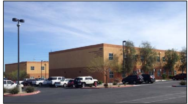
13. McLeod Complex Building 1 (Student Services Division )
